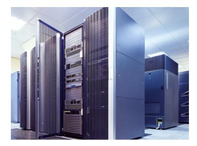
The unassuming exterior houses a proprietary free-air/CRAC cooling system. This technology gives DC5 a real world PUE of 1.2, making it one of the most efficient data centres in the Central London metro market.
